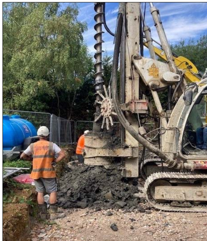
Pile driving on site at Crofts Court
