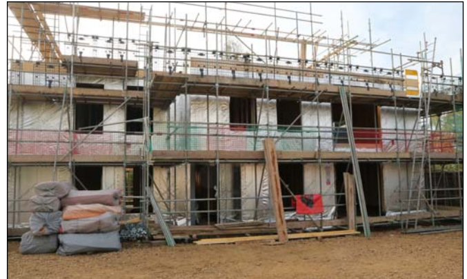
Timber frame progress late October 2022
