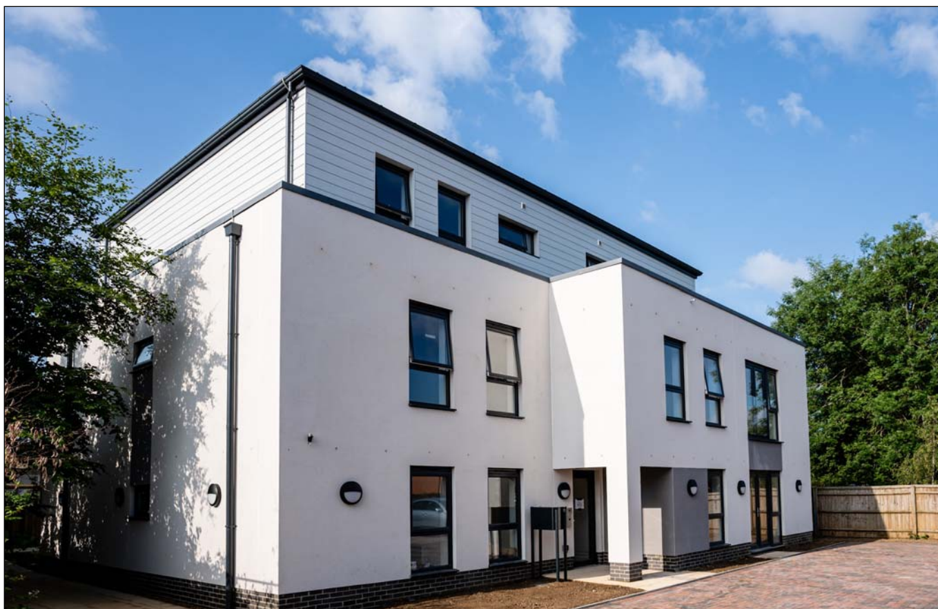
Crofts Court – the finished building in July 2023
