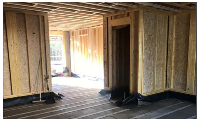
November 2022 internal progress
